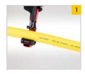
**D1.** Cut tubing at required length with a tubing cutter between two corrugations. Tighten roller pressure slightly after each revolution. If the end of the tube is not smooth and there are burrs please cut tubing again.
